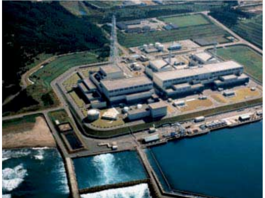
Kashiwazaki-Kariwa Nuclear Power Station – the largest nuclear power station in the world is operated by Tokyo Electric Power Co., USEC's biggest customer. The seven boiling water reactors there generate 8,212 megawatts of electricity.
